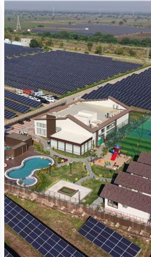
Iconic Solar Park Solarism , Jambusar - Bharuch Rd, Sudi, Ranada, Gujarat 392025
